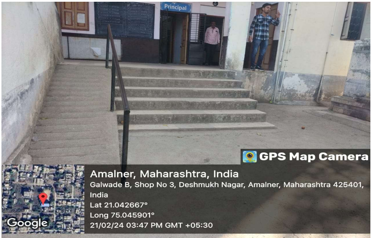
Ramp For Differently Abled Students
